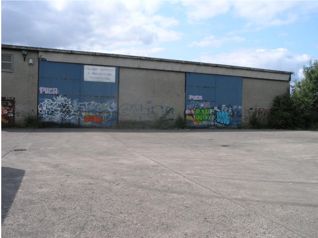
Figure 13.10: Vacant building and car-park on east side of development
